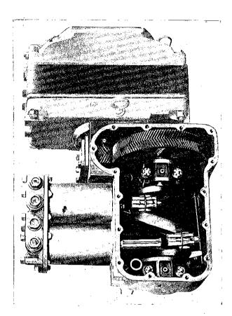
The air valves, four in number (one suction and one discharge valve for each cylinder) are located close to the cylinder compression space to reduce valve clearance. Placed vertically, they close by gravity, no valve springs being required. The valve stops are designed to reduce clearance and prevent sluggish action of the valve.
